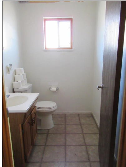
13.0 Item 3(Picture) - The maneuvering clearance in front of the water closet is not compliant.
