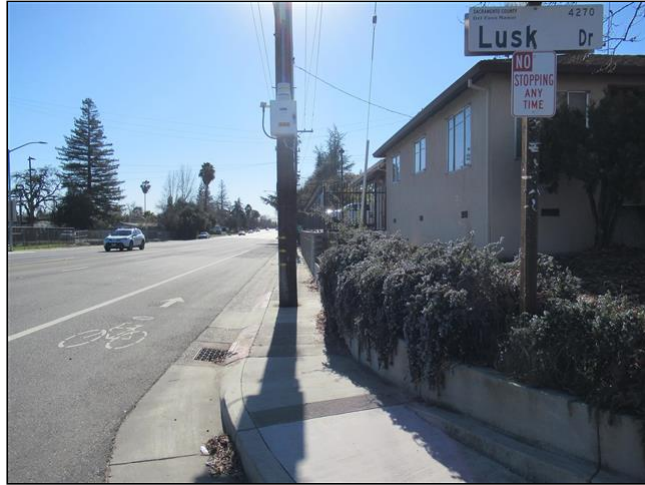
2.0 Item 3(Picture) - View showing inaccessible public sidewalk due to the placement of utility poles.
