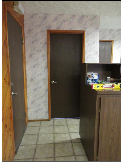
13.0 Item 1(Picture) - The entrance to the restroom is not compliant.
