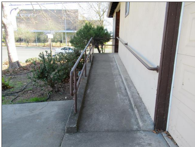
5.0 Item 4(Picture) - The wall brackets that secure the right handrail are not compliant.
