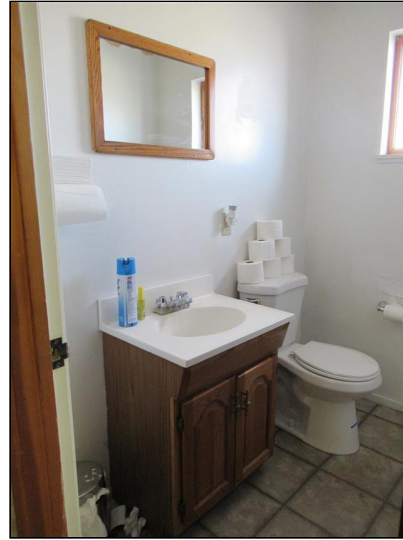
13.0 Item 2(Picture) - All elements within the restroom are not compliant.
