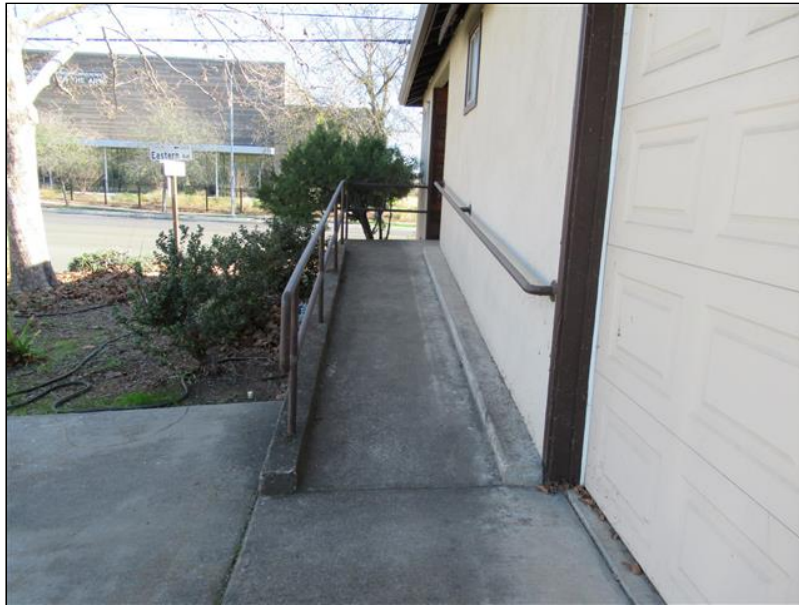
5.0 Item 1(Picture) - The ramp is not compliant.
