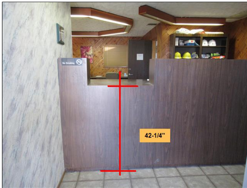
10.0 Item 1(Picture) - The transaction counter is not accessible.
