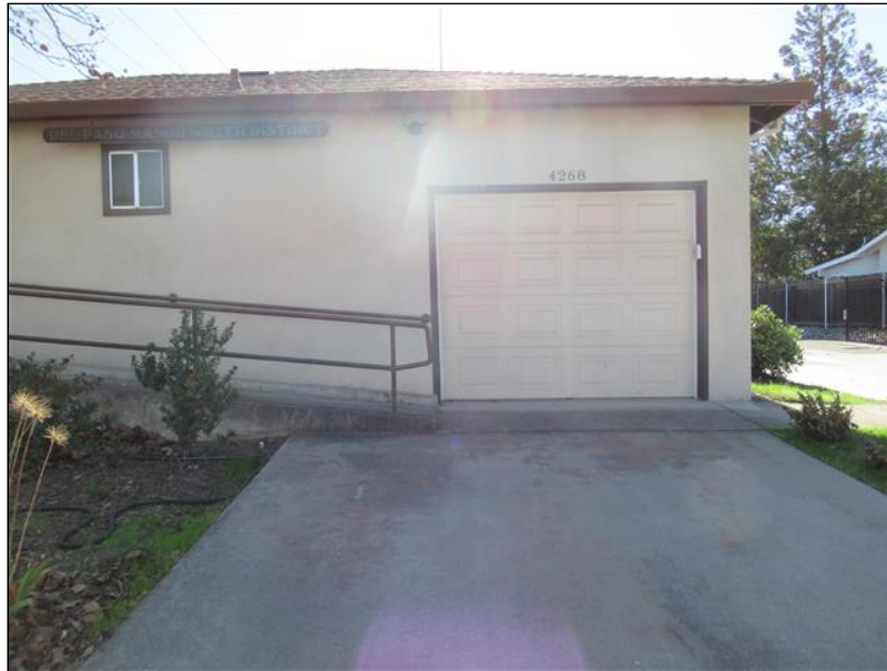
5.0 Item 3(Picture) - The bottom handrail extensions and bottom landing are not compliant.
