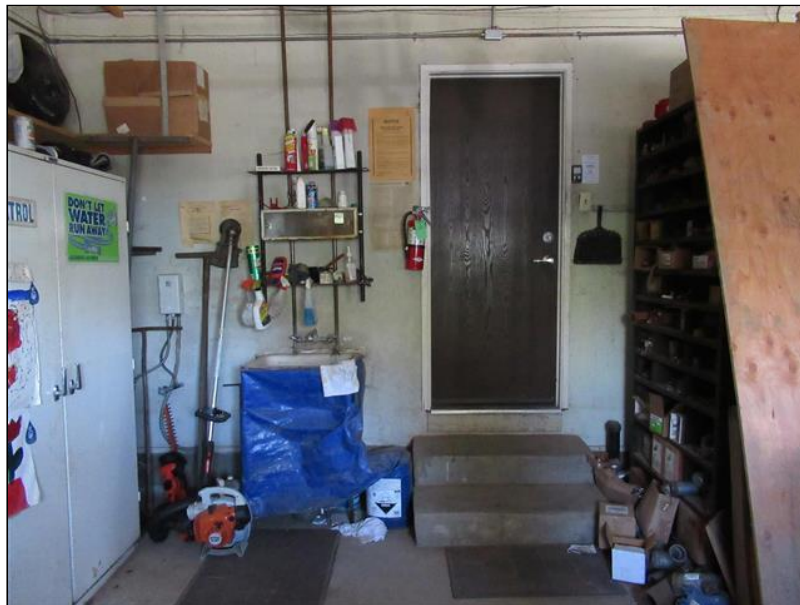
8.0 Item 2(Picture) - A door landing is required. Compliant stairs, handrails and possible guards are required.
