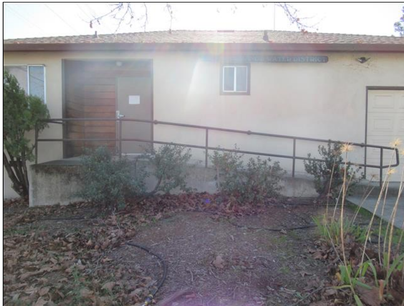
5.0 Item 2(Picture) - Front view of non-compliant ramp.
