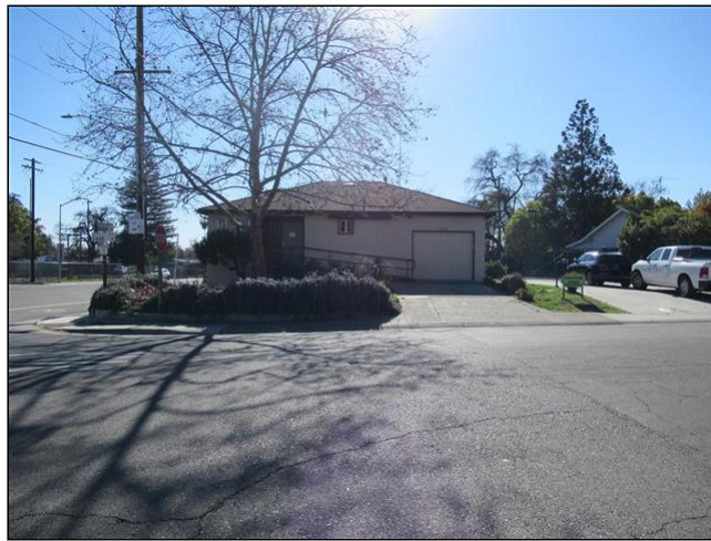
2.0 Item 1(Picture) - View showing public sidewalk and curb ramp.
