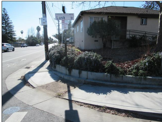
2.0 Item 2(Picture) - Close-up view of curb ramp at the corner of Eastern Ave. & Lusk Ave.
