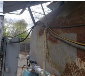
• The path of travel is restricted and also has overhead hazard. The second photo shows that there is no room to travel on other side of tank.
