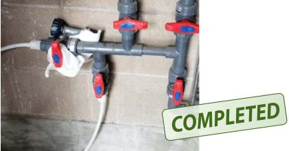
• Chemical degas pump discharges into an open bucket.
