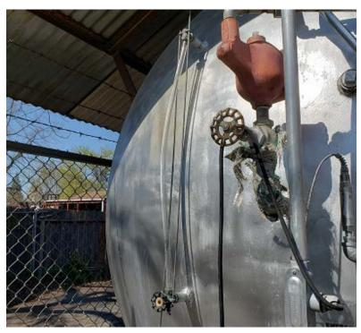
• The eyewash station position introduces potential hazards. There are tank appurtenances that could cause injury in the event an operator is in need of the eyewash station.
