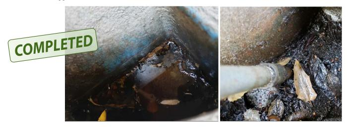
• Pump base seal is separating. When the well turns off, contaminants could potentially be sucked into the aquifer.
