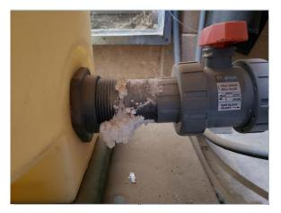
• Sodium Hypochlorite Tank will drain if ball valve opens, fails, or breaks off.
