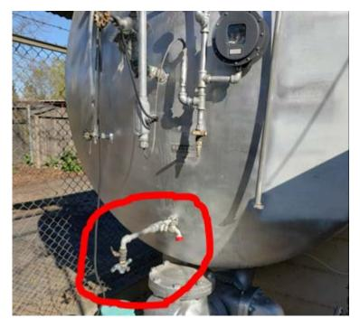
• Electrical conduit and equipment sealed with tape rather than the correct means. Electrical cables are strung across the tank and draped in the air presenting additional hazards.
