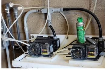
• Chemical pumps have leaks and build up. Rags are used to absorb chemical drips.
