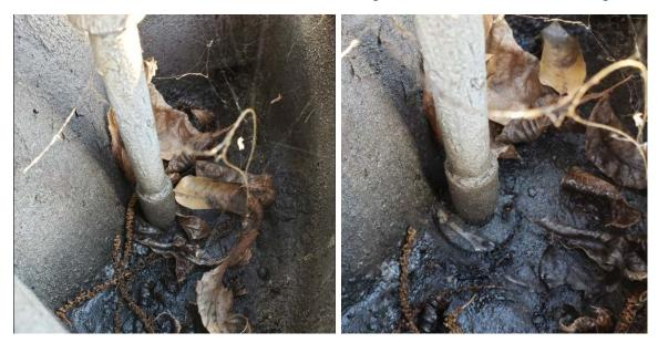
• Chemical injection was isolated (off) at the injection assembly. SSWD staff went to restore the chemical injection into service and found the assembly broken in multiple locations. SSWD made immediate repairs. Well #2 has history of raw water Bac-T positive samples and DDW allowed DPMWD to keep it in service only if continuously chlorinated.
