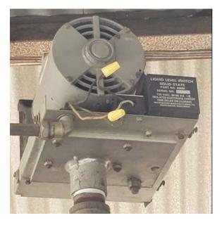
• Electrical LB junction box is secured with Duct Tape instead of the appropriate two screws holding the plate and gasket to seal against weather conditions.
